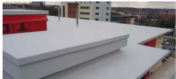
Completed warm roof suitable for occasional foot traffic.
