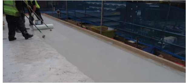
Application of waterproofing direct to primed insulation.
