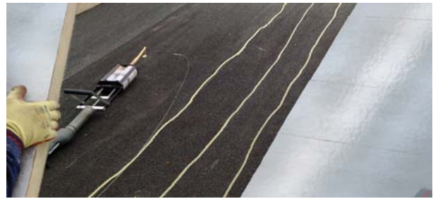
New insulation provided. Adhesive or mechanical fix.
